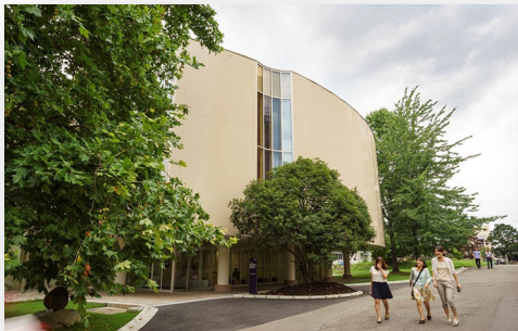
▲ Seiryō Kaikan exterior
